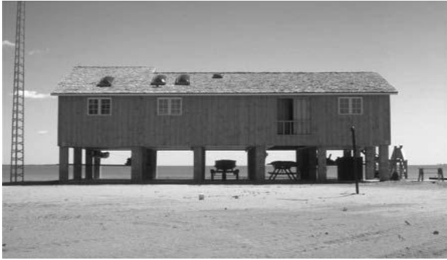
Figure 3.3: Flood proofed dwelling
