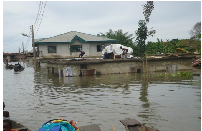
Figure 3.2: Submerged Buildings In Ogbaru L.G.A
