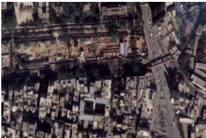
Fig. 7: Air monitoring station (BRRC, Farmgate, Dhaka)
