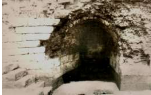
pl. 31. A part of the staircase on the northern wall
