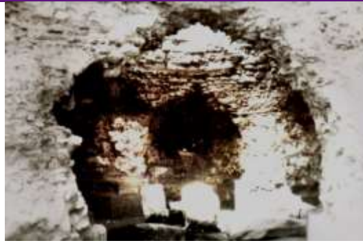
pl. 29. Entrance to the North western Tower
