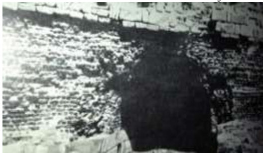
pl. 10. An embrasure and shows the places of the stones removed by the people
