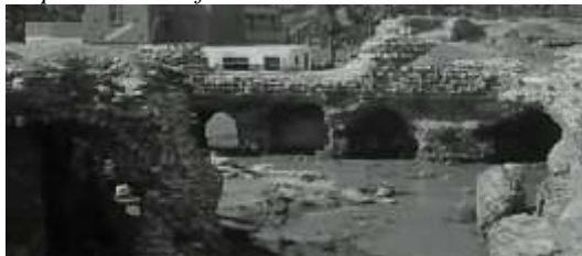
pl. 7. The remains of the fences from the inside and the Keep
