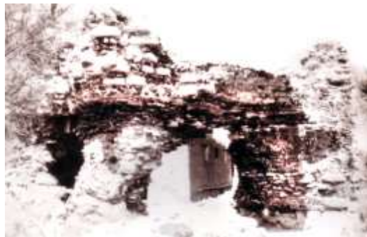
pl. 20. South eastern tower
