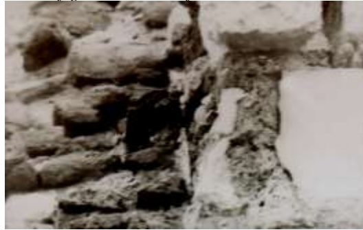
pl. 22. The corridor that used to represent the second floor of the castle walls
