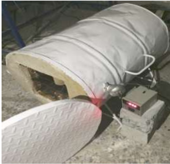
Fig. 2.3: The installation of grate and instruments
