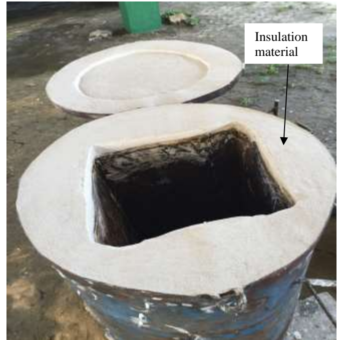
Fig. 2.2: Instalment of the insulation material
