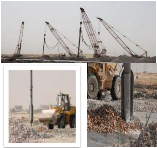
Figure 6: Installation of stone columns on-site
