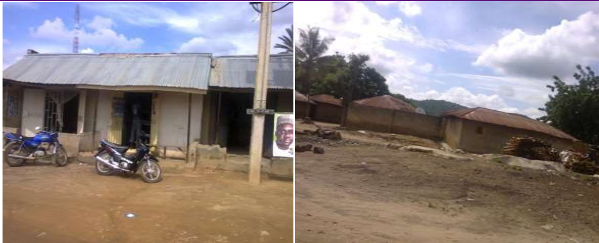
Plate II: Showing some of the building with zinc corrugated roofing sheet
