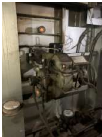
Figure 2.2 Gun type burner
