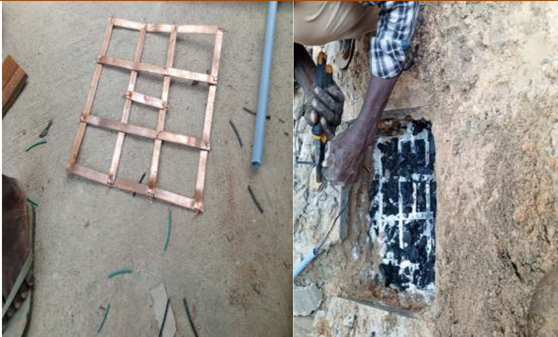
Plate 4: Construction and Installation of earth mat
