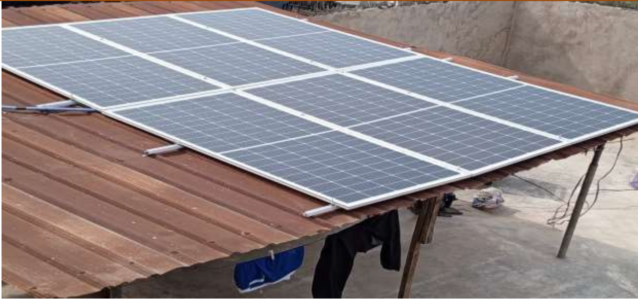
Plate 2: Mounted panel on the mounting rays
