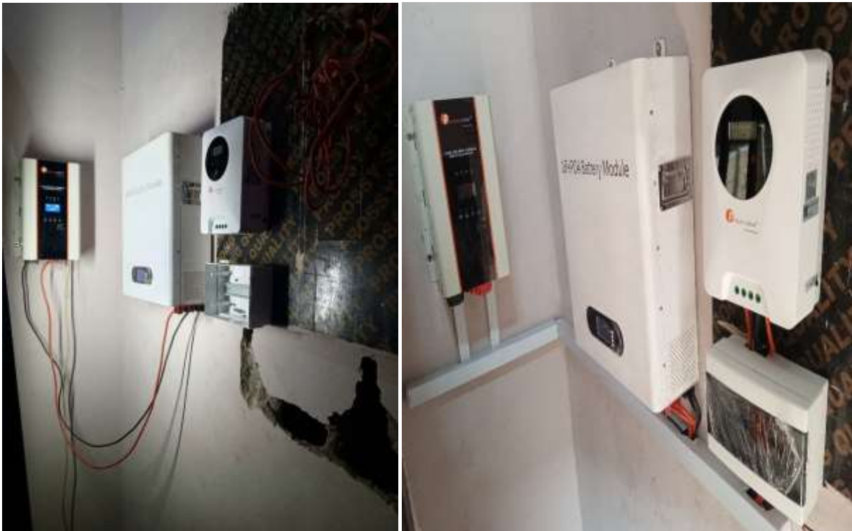
Plate 3: Installation of Battery, Inverter, Controller, and Service box in Progress
