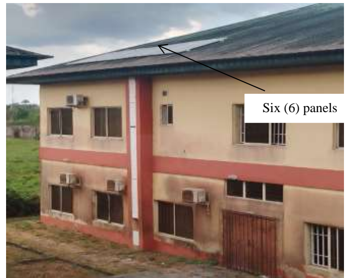
Plate 1: Installation of the solar panels
