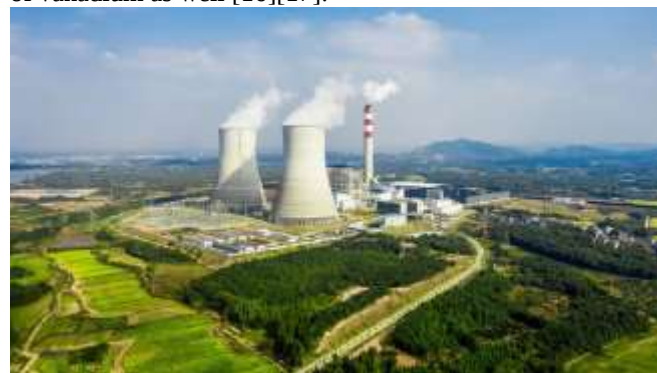
Figure 1.2 Thermal power plant
